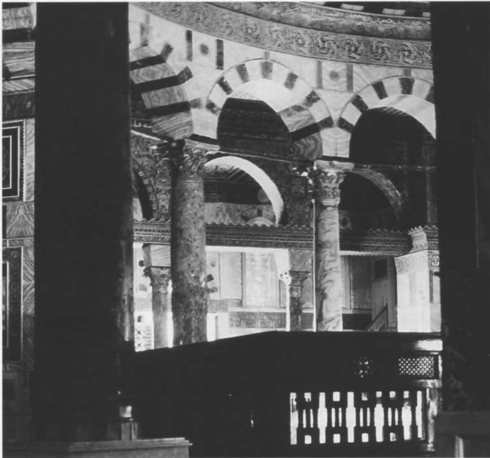
Figure 13. Dome of the Rock, view from edge of inner ambulatory across the rock showing twist to colonnade.
